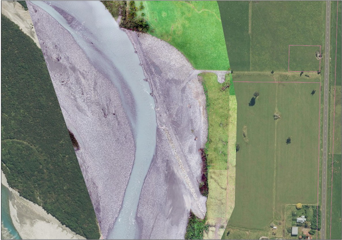
Image 1: Aerial footage taken on the 28 th of May 2022. Note the erosion occurring between the spurs. This erosion had been repaired by the landowner before the stopbank failure.
