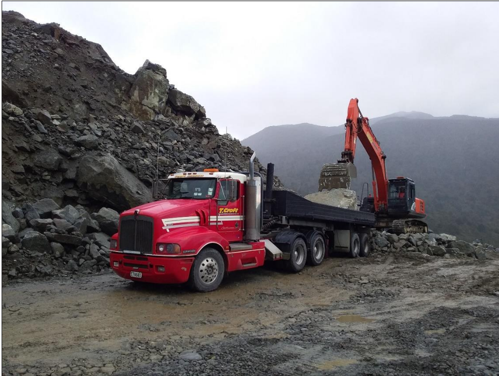
Figure 8 Loading out of armour rock (2Ton)
