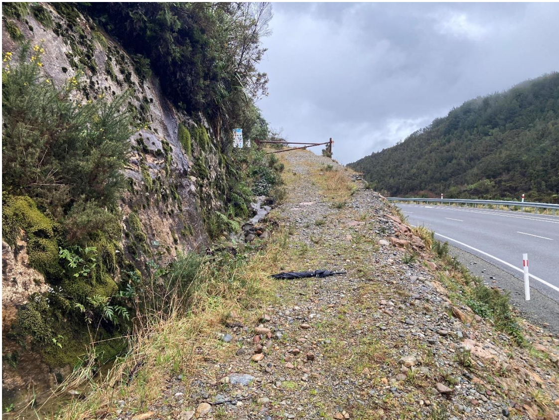
Plate 6. Pinch point at intersection of accessway and public road. Usable width here is around 3 m if the water table on the left is temporarily infilled.
