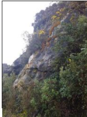
Figure 2 Fractured rock to the left of the access road
