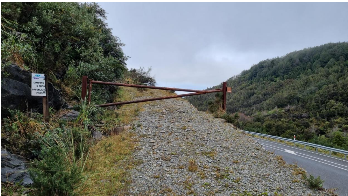
Figure 3 2022 Access Road has been narrowed with the Roa Road improvements
