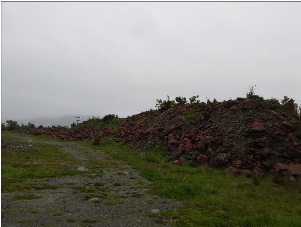
Figure 13 Piles of stock and/or waste are throughout the quarry site
