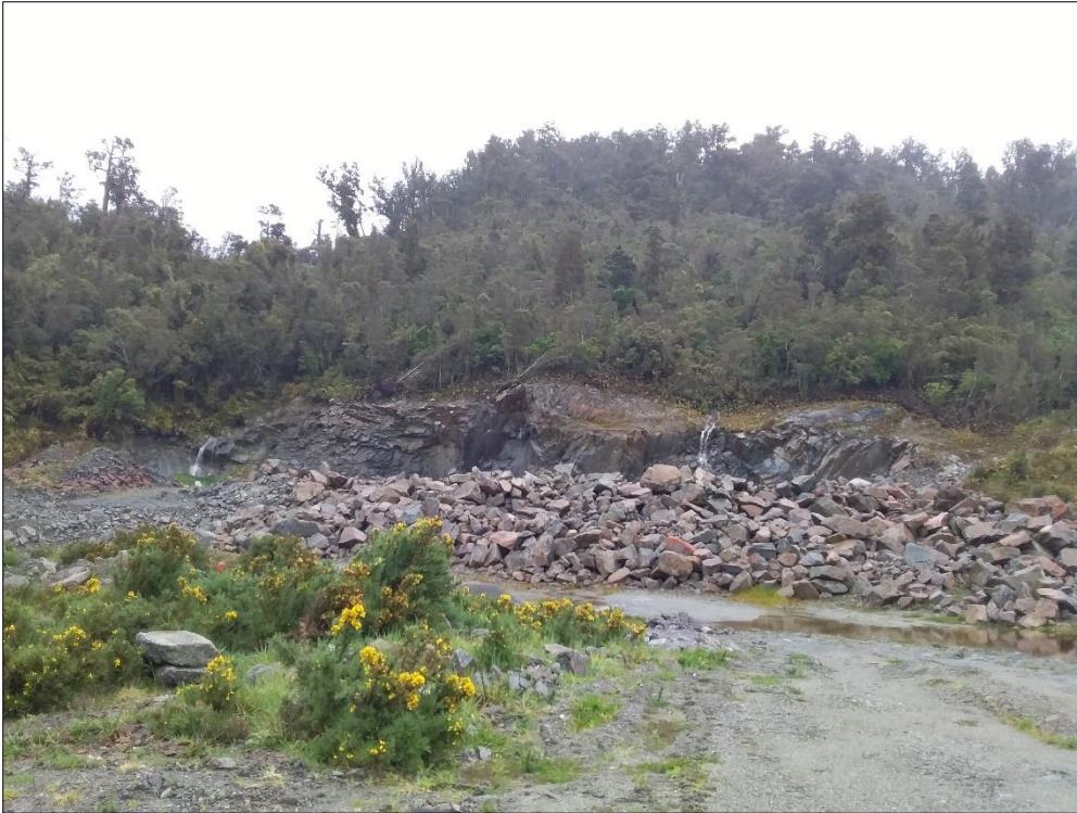
Figure 14 Benches are clearly visible with water entering through the face.
